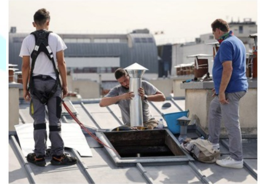
In process: A roofer and zinc worker on the roof of a building in Paris. AFP
