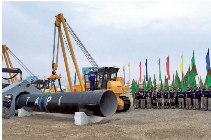
Slow progress: Work on the pipeline has been delayed by security issues in Afghanistan. FILE PHOTO
