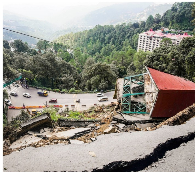
A road damaged by a landslide triggered by heavy rain at Baluganj in Shimla on August 21. Most regions of India now expect weather extremes in all seasons. PTI
