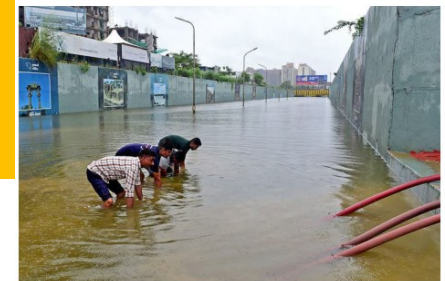
Emergency services personnel work on removing water from a flooded underpass on the outskirts of Ahmedabad. AFP
