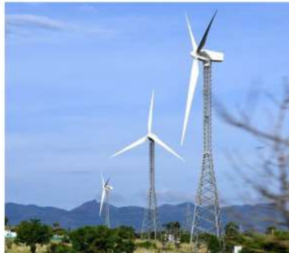
Powerhouse: Wind turbines along the Kadayanalur-Tenkasi highway in Tamil Nadu. JITHUNISAKUNGAN
