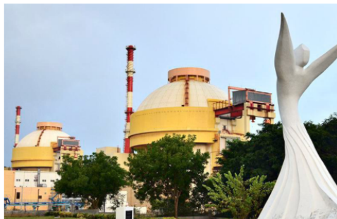
Joint effort: Rosatom, the only foreign nuclear operator in India, is involved in the Kudankulam Nuclear Power Plant in Tamil Nadu.
