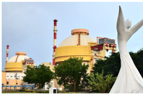
Joint effort: Rosatom, the only foreign nuclear operator in India, is involved in the Kudankulam Nuclear Power Plant in Tamil Nadu.
