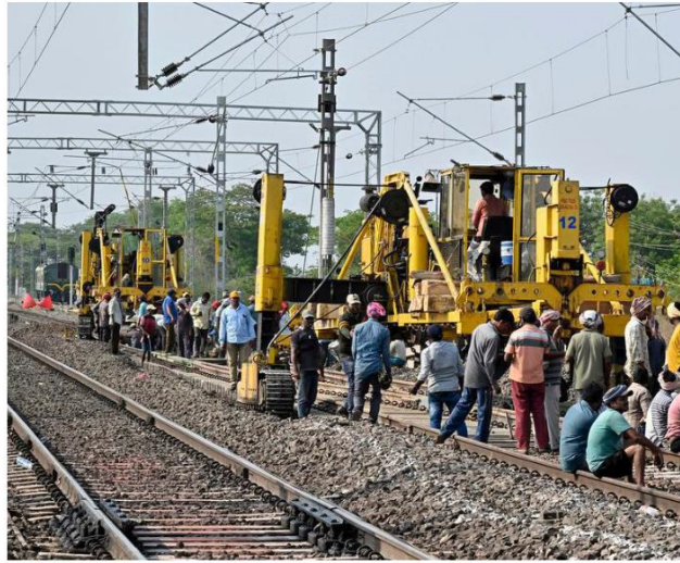
Not enough: A group of workers and officers of the South Central Railway working on the electrical lines between Vijayawada and Kazipet junction in the Andhra-Telangana border area in 2024. G.N. RAO
